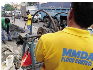
Cleaning of Manholes
